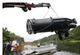
The destratification devices are composed of three pipes that entrain and direct the water horizontally. Images Andy Bruere and Hans Burggraaf.
