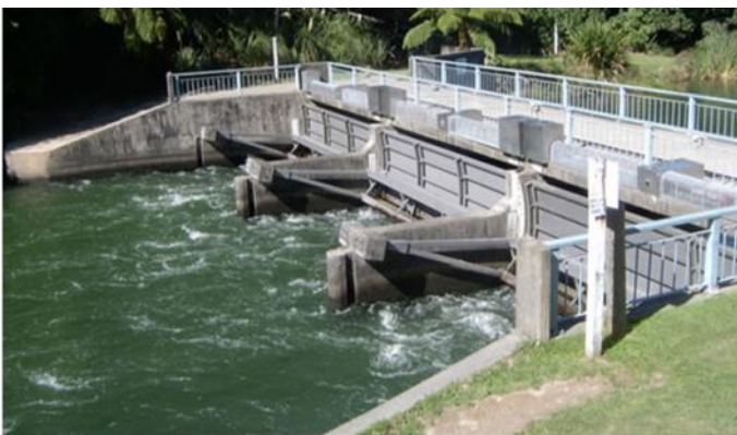
Okere flood gates (Photo: Environment Bay of Plenty)
