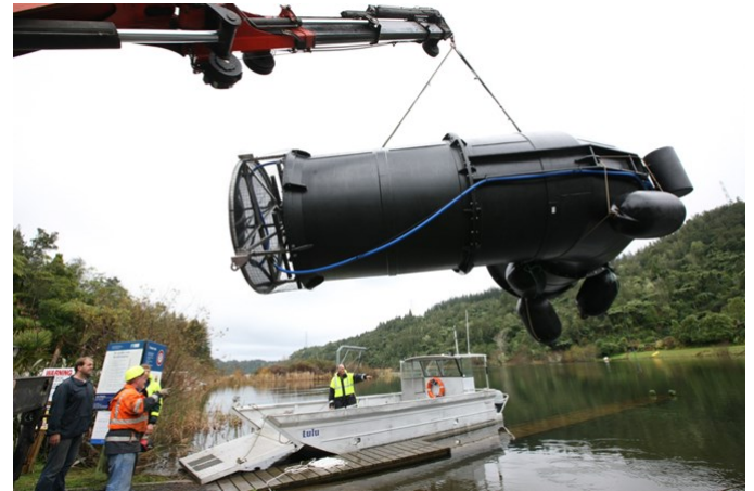
Figure 3. A section of a destratification device prior to installation in Lake Rotoehu. Image: Andy Bruere
